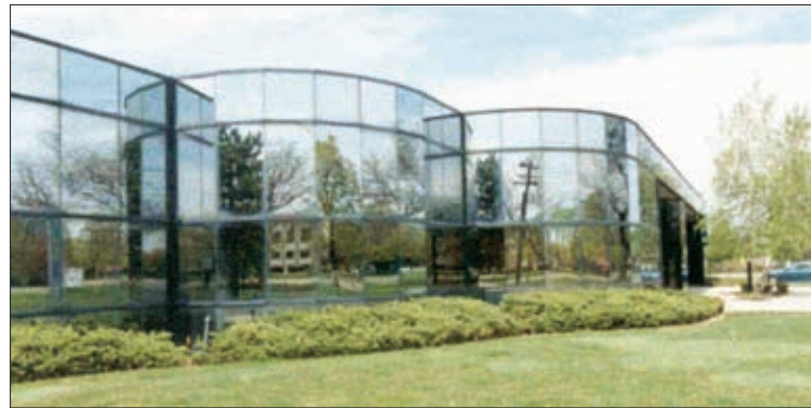
532 Broadhollow Road (above) and the atrium at Melville Corporate Center III (right).
